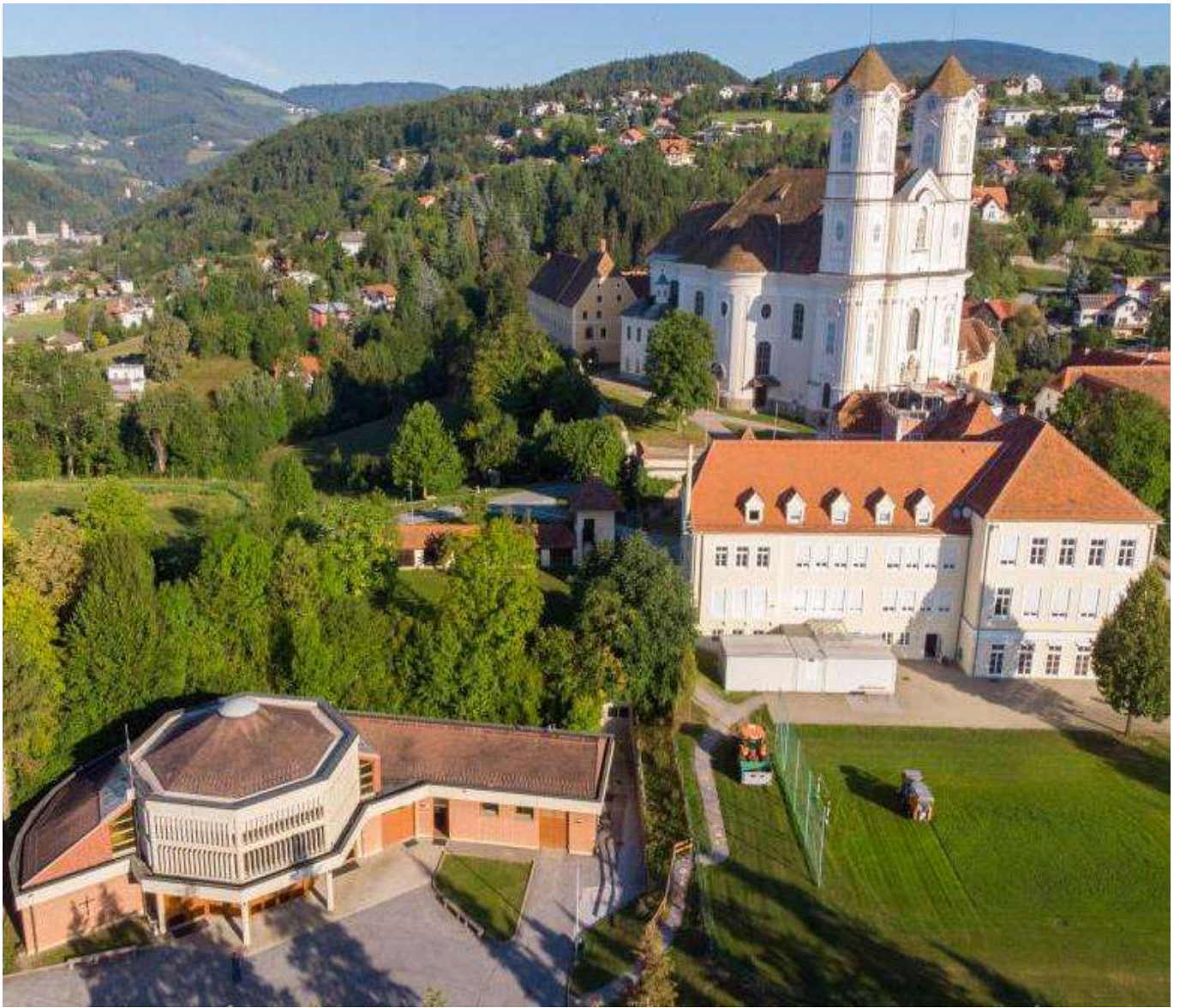
View of the existing biomass heating plant in the Weizberg to the north
